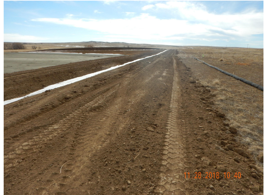
Photo 4. Photo taken from the northwestern perimeter of the location, facing South. Filtrexx wattle BMP has been installed throughout the entire perimeter of the location in conjunction with other BMPs.
