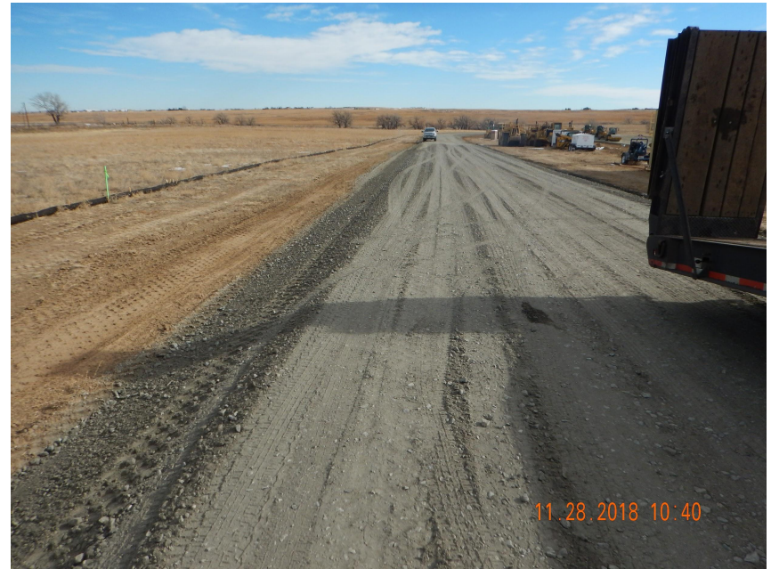
Photo 2. Photo taken from the entrance of the location, facing East. Photo illustrates the Operator is in process of stabilizing the main access road with road base. Filtrexx wattle BMP was observed throughout the entire perimeter of the location in conjunction with other BMPs. Note: Operator has stored equipment between the main access road and the location. Operator is responsible for reclaiming all disturbances associated with oil and gas disturbance.
