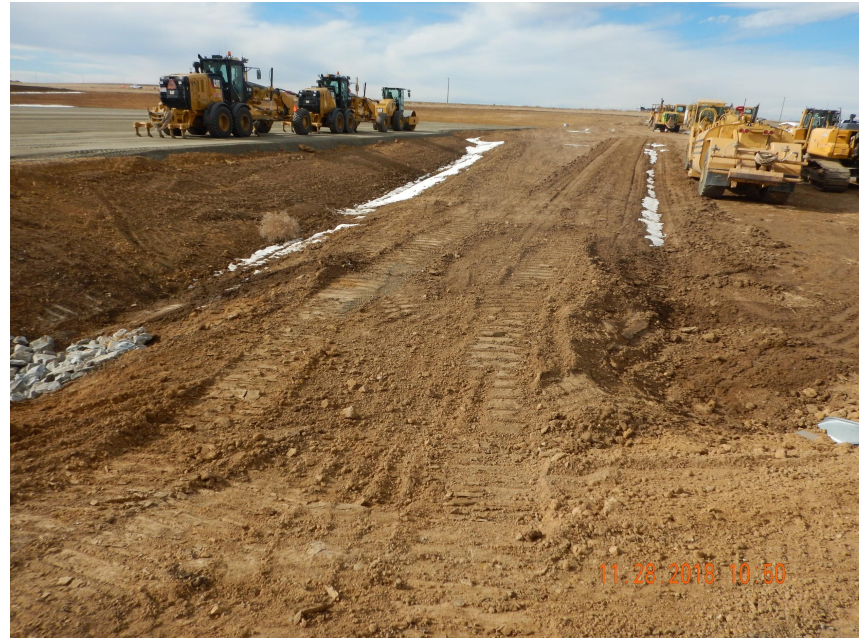
Photo 10. Photo taken from the northern location, facing West. Photo illustrates two sets of ditch BMPs which are directed to the stabilized outlet.
