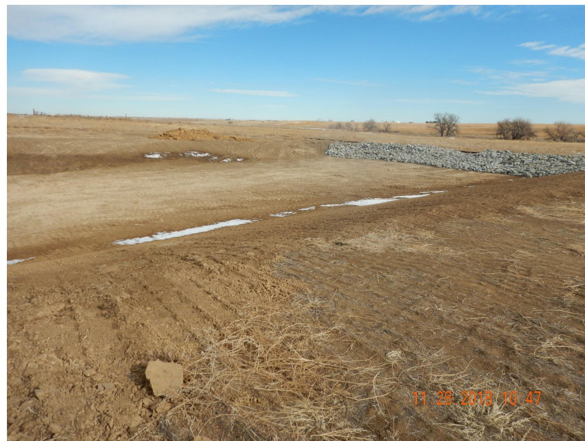
Photo 8. Photo taken from the northeastern perimeter of the location, facing Northeast. Photo illustrates a sediment trap installed with a stabilized outlet.
