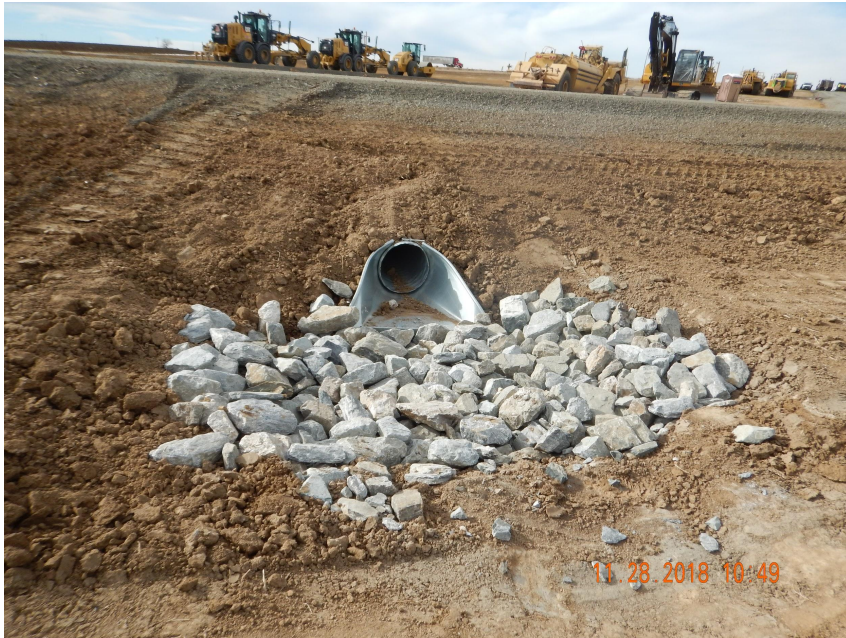
Photo 9. Photo taken from the outlet of a culvert, facing West. Stormwater is directed to the stabilized sediment trap.
