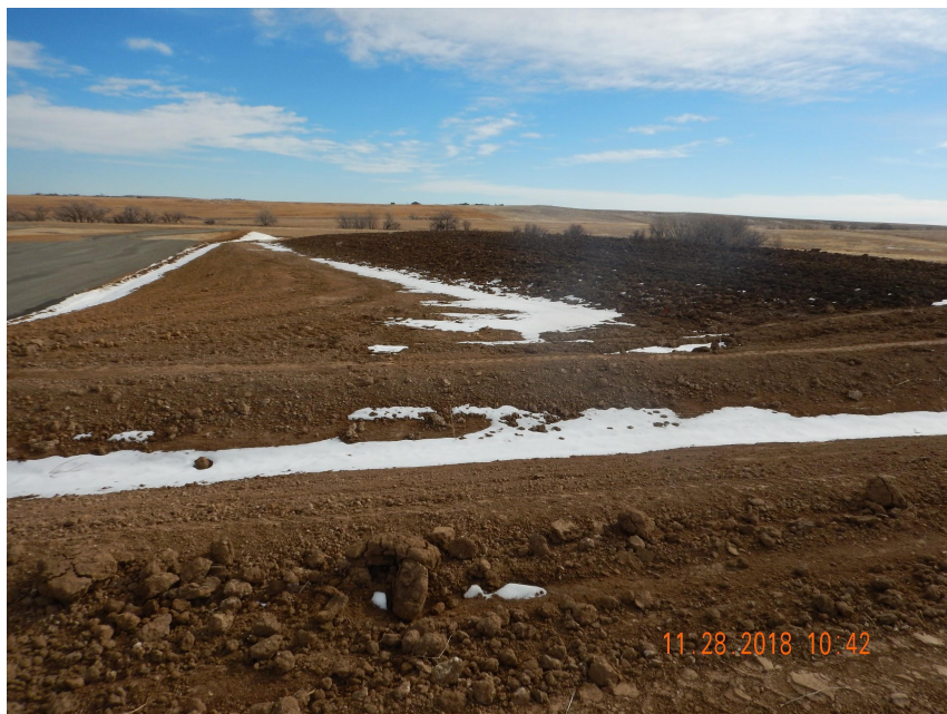
Photo 7. Photo taken from the southwestern perimeter of the location, facing East. Photo illustrates the topsoil stockpile that has been temporarily stabilized with equipment tracking.
