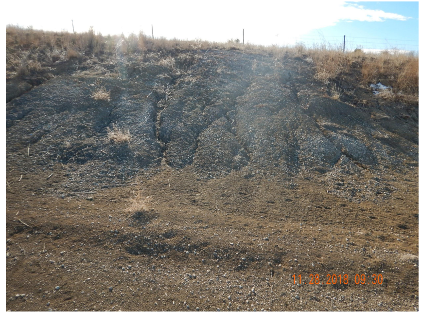
Photo 2. Photo taken from the southwestern cut slope, facing South. Photo illustrates an unstabilized cut slope with the evidence of rill erosion. The entire southern cut slope has not been properly stabilized. This location is not in compliance with Rule 1002 standards.
