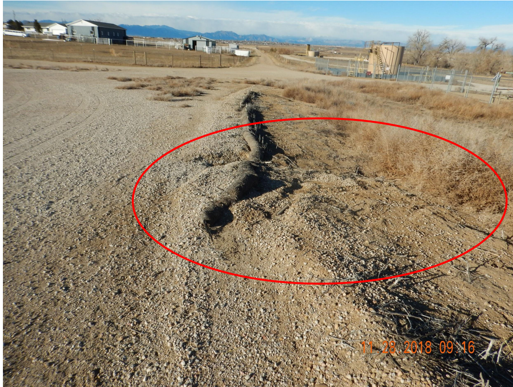
Photo 5. Photo taken from the northwestern location, facing West. Photo illustrates stormwater erosion discharging off location. This location is not in compliance with Rule 1002 standards. Note: Weeds (Kochia) were observed along the northern and northwestern perimeter of the location that have not been managed.
