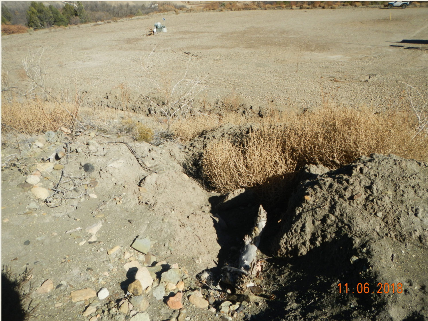
Photo 11. View of erosional channel forming from stormwater run-on within the western cut-slope.
