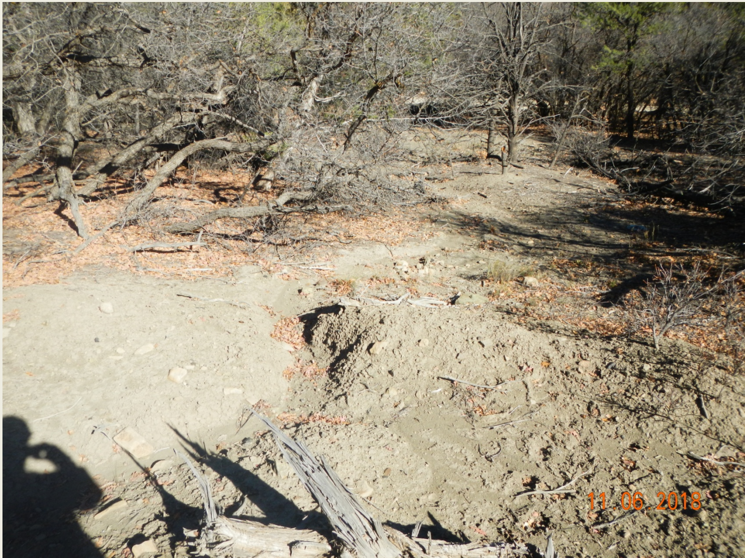
Photo 7. View of unstabilized soils, erosional channel approximately 2 feet wide and 1.5 feet deep, and sediment deposition/transport in the northwestern project area.
