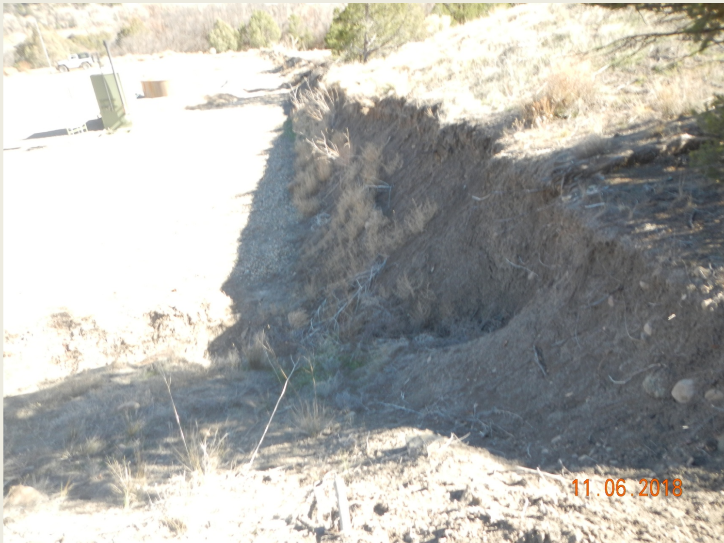
Photo 12. View of the southern project area from the southwestern corner facing eastward. Cut-slope is not stabilized.
