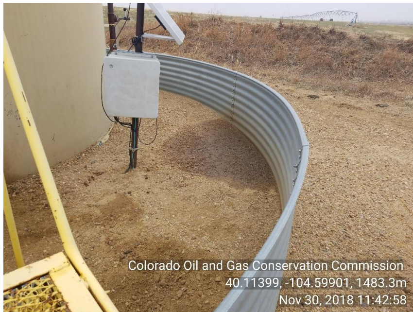
Photo 3 Stained soil in containment next to crude oil tank
