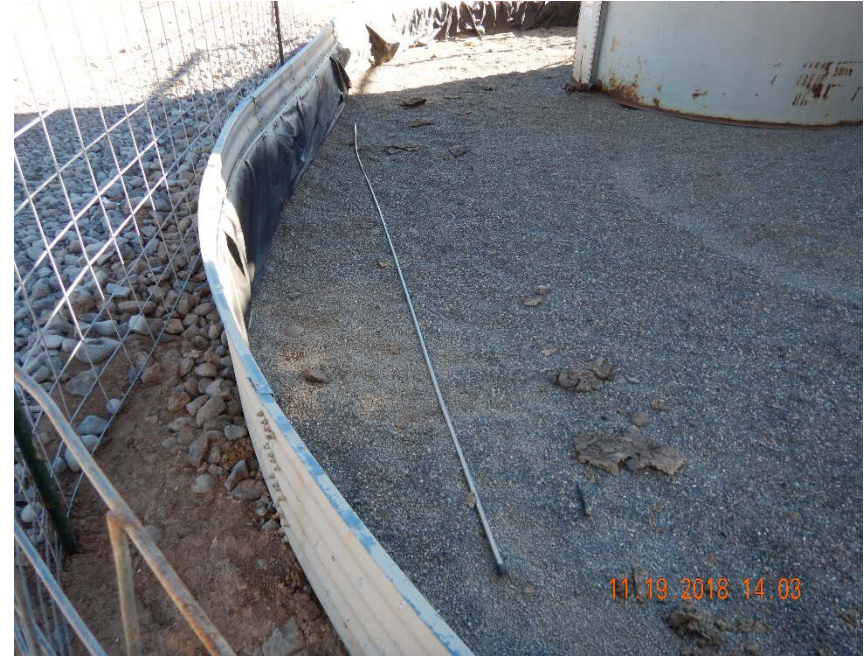
Photo #10 – ¼" Stainless steel line stored inside of tank battery SPCC of smaller tank battery. COGCC contacted operator on 11/21/2018 and instructed to remove unused equipment from SPCC.
