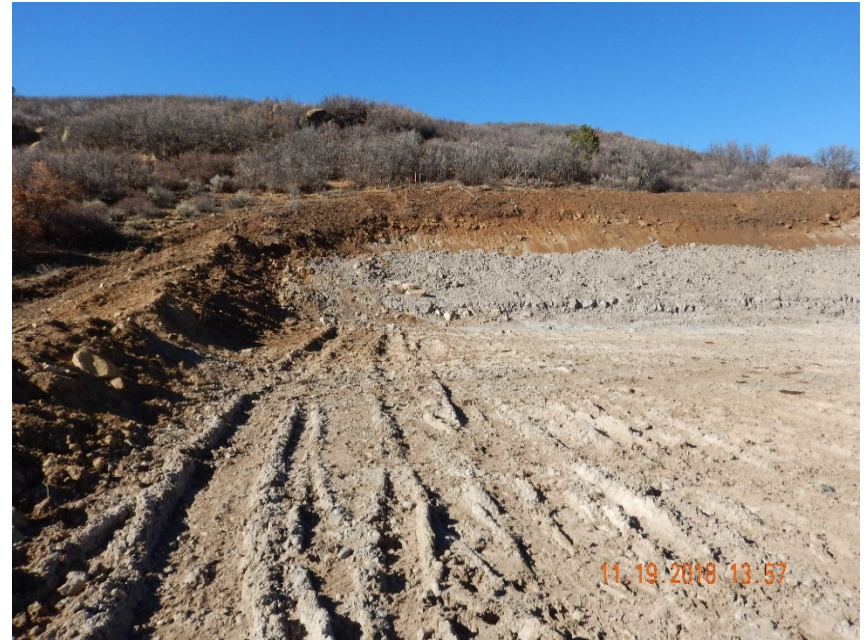
Photo #4 – Location of Spill/Release ID #456712. Note cuttings stockpile lacks stormwater control BMPs.
