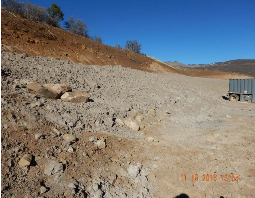
Photo #5 – View of cuttings stockpile at southwest corner of pad. Note absence of stormwater control BMPs around cuttings stockpile.
