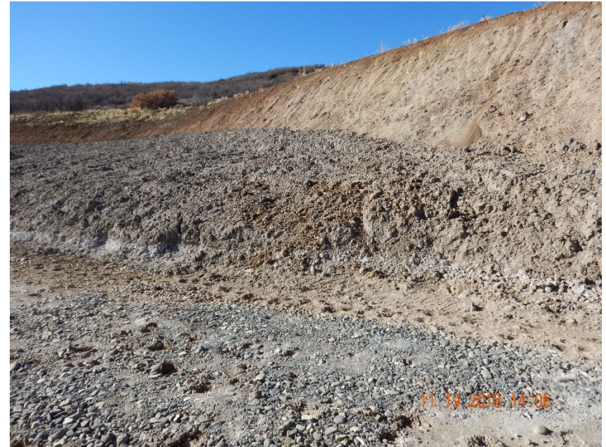
Photo #6 – View of cuttings stockpile along northwest side of pad. Note absence of stormwater control BMPs to prevent stormwater runoff and sediment transport from cuttings stockpile.
