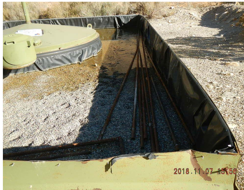
Joints of pipe stored in secondary containment berm.
