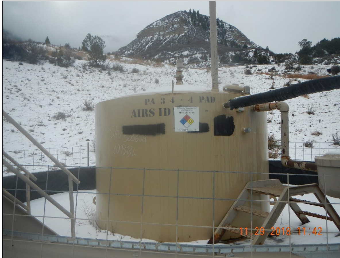
Wrong well/pad name on tank. Capacity is fading on label.
