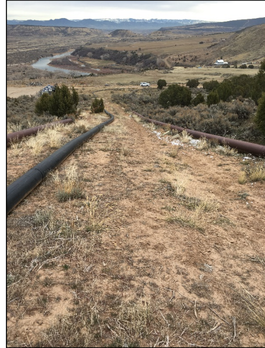
Poly and steel flowline from pit towards location
