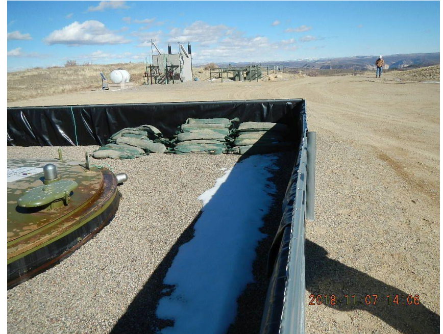
Sandbags stored in secondary containment berm.
