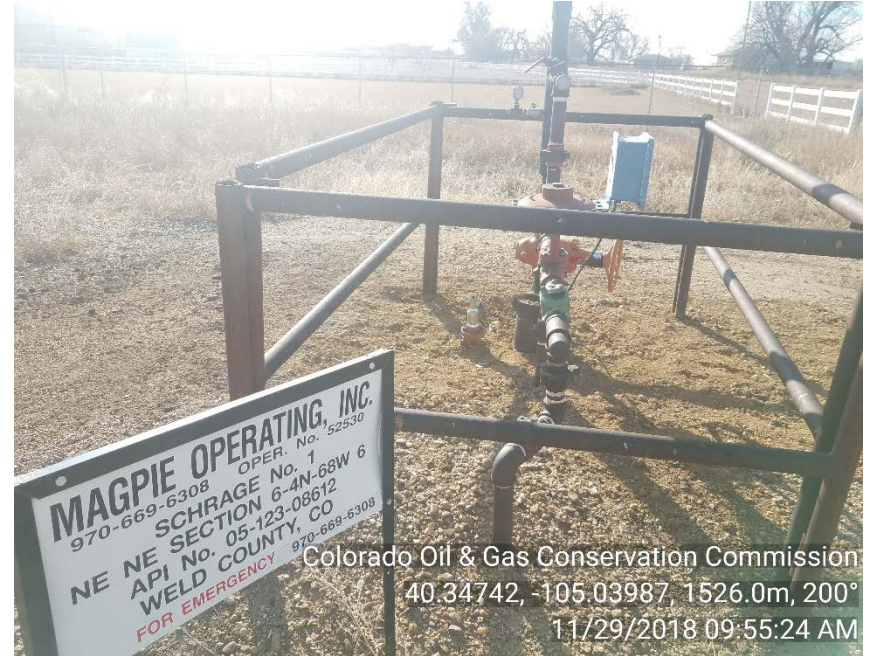
Wellhead and Bradenhead valve on 11/29/18
