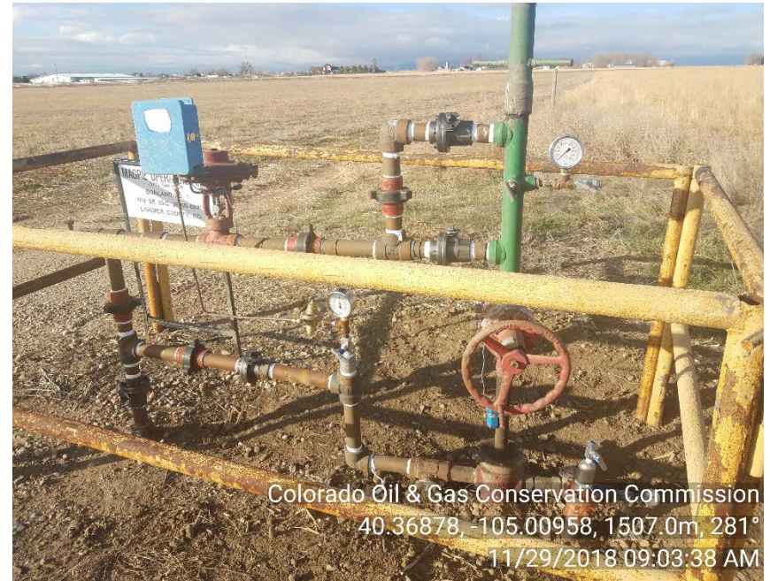
Bradenhead valve on 11/29/18
