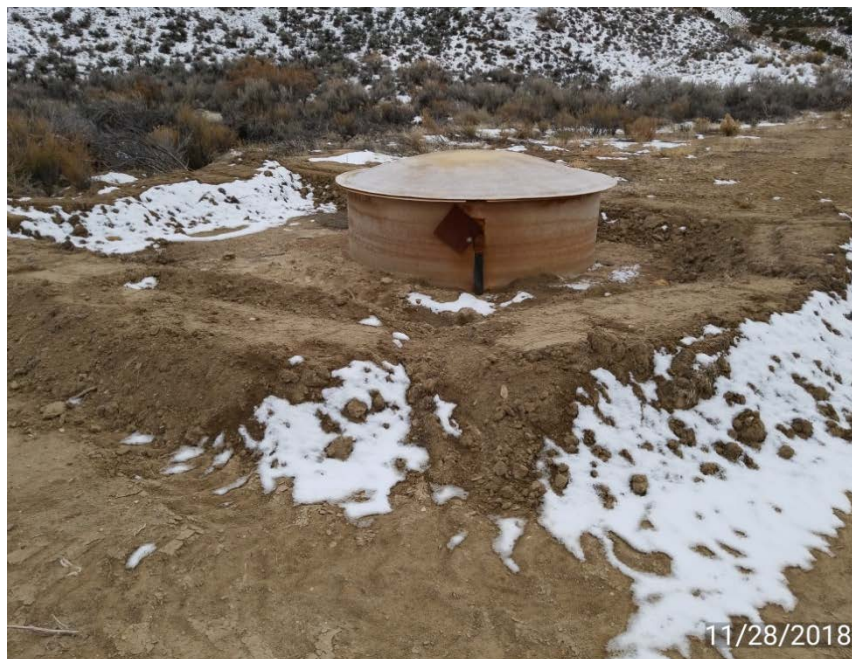
Photo 1. Berm added around tank.
