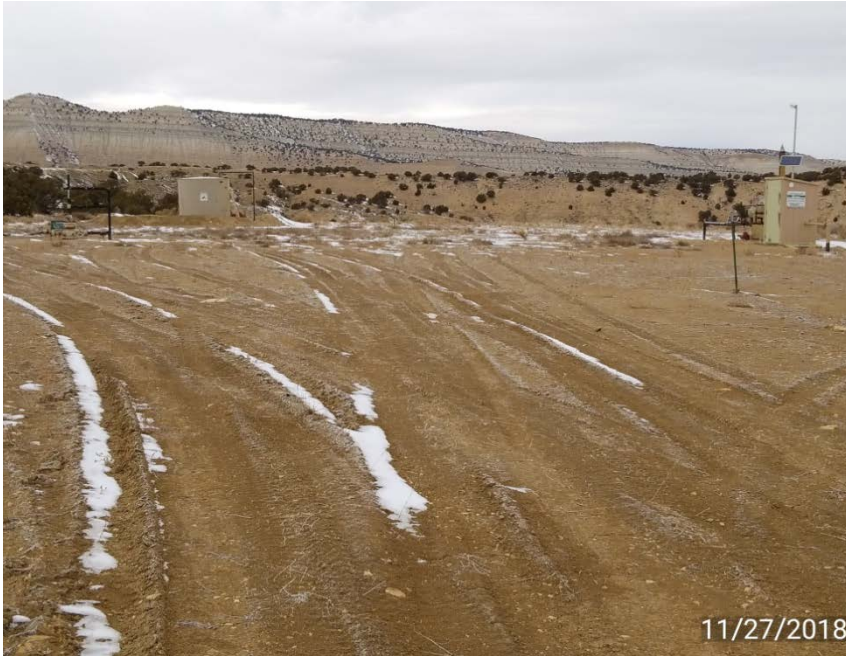
Photo 1. Location looking west.
