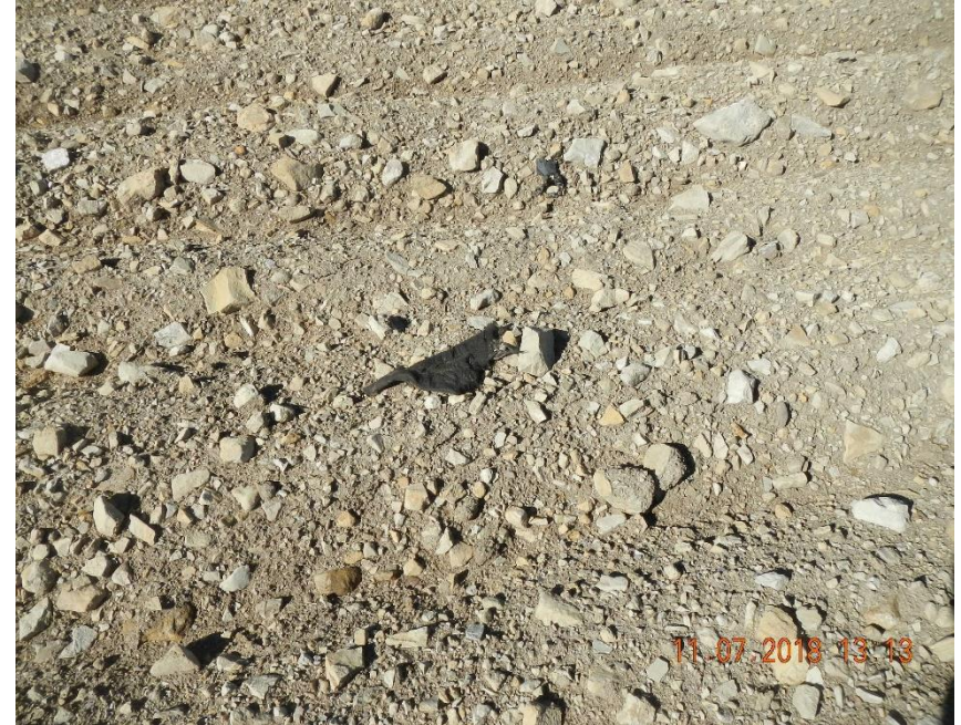
Remove liner pieces as they become exposed in landfarmed material.
