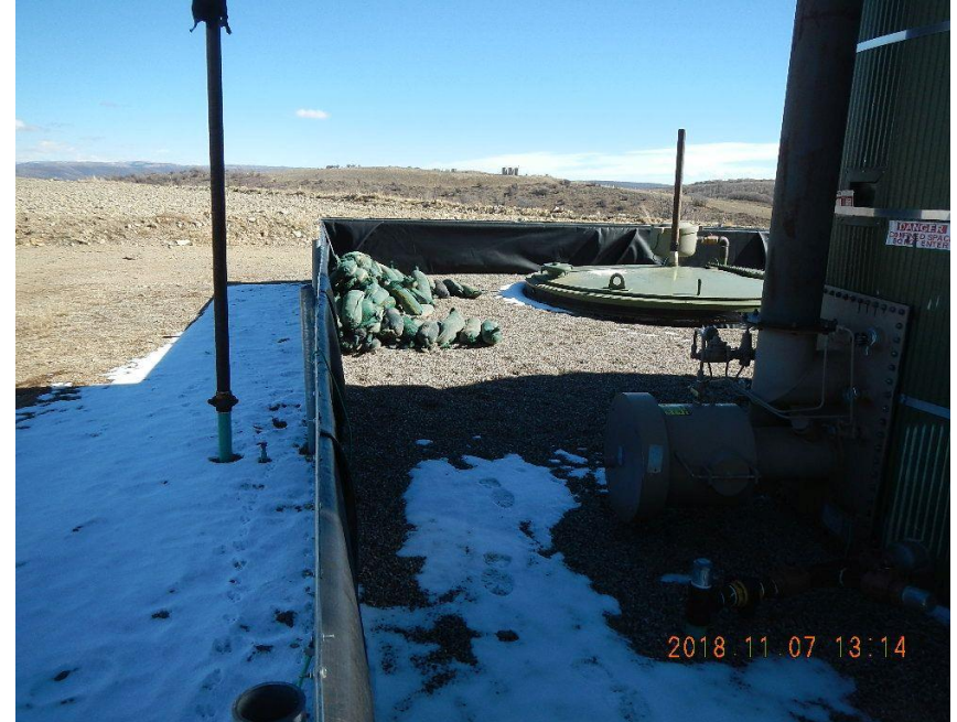
Sandbags stored in secondary containment berm.
