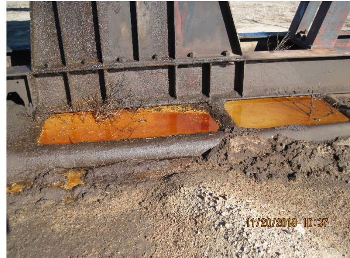
2. Oily water in unit base, south side of unit
