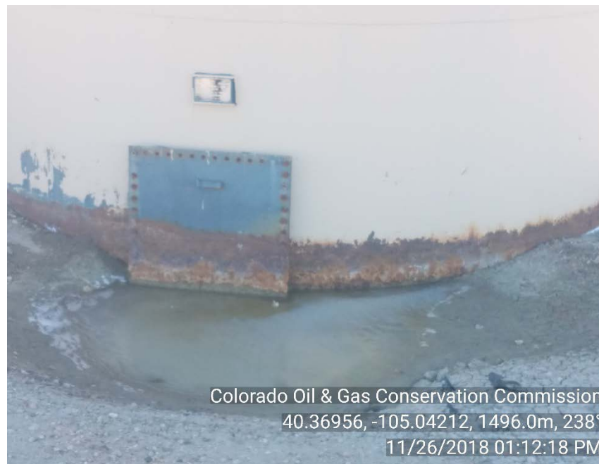
Rear of produced water tank showing clean out plate and corrosion
