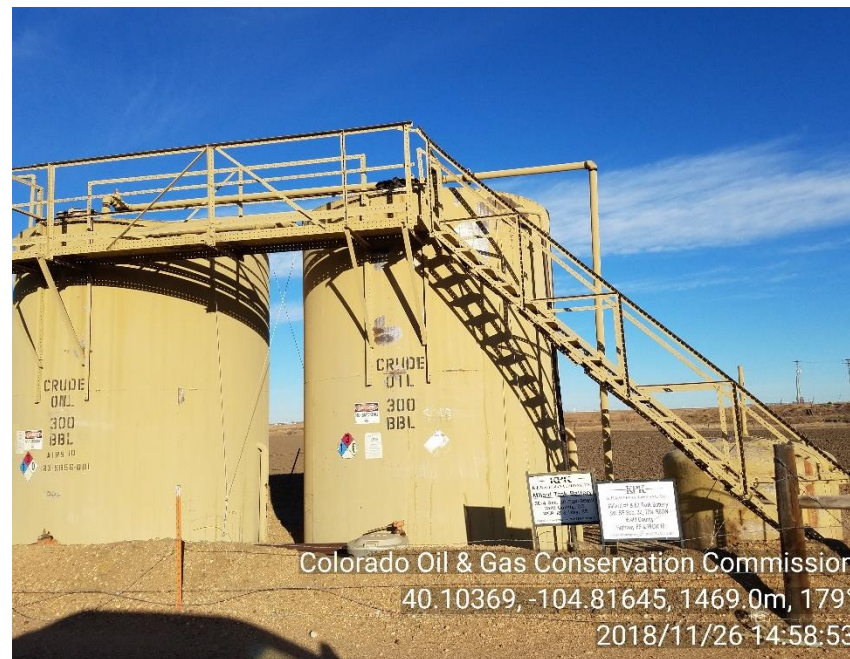
PHOTO 2: TANK BATTERY
