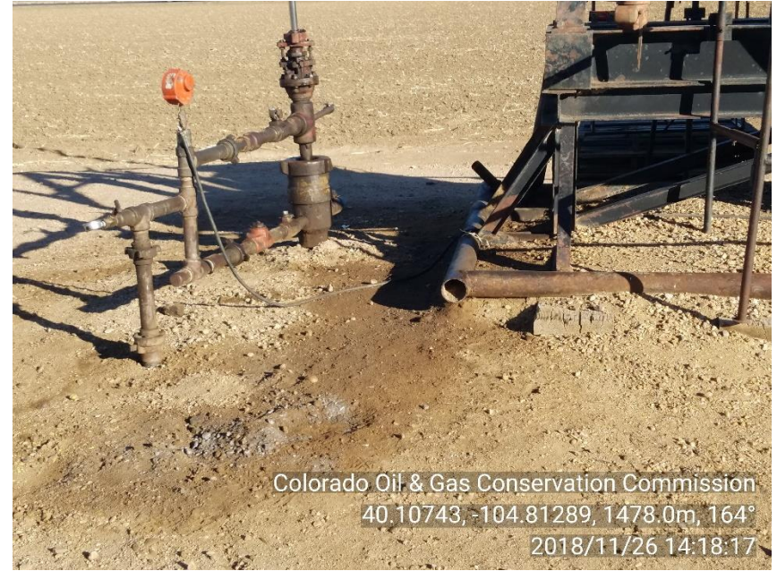
PHOTO 2: STAINED SOIL AROUND WELLHEAD
