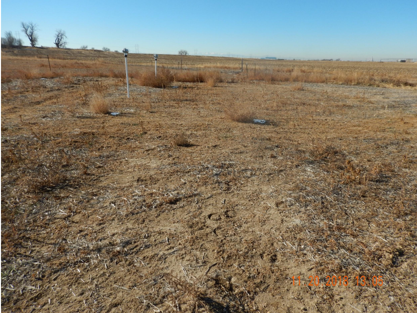
Photo 1. Photo taken from the battery location (non-cropland), facing West. Appears the Operator has started to perform final reclamation activities but Remediation Project #10881 is still active. Operator shall continue to monitor and control weeds and stormwater until the location meets Rule 1004 standards during the remediation process. Well location and access road were fallow cropland so a future final reclamation inspection will be conducted.
