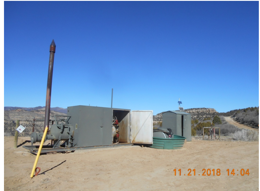
Separator, Meter housing and Secondary chemical storage
