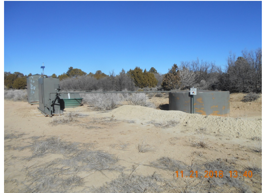
Separator, Meter housing and Tank battery
