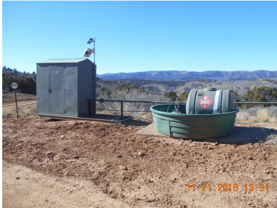
Meter housing and Secondary containment of chemicals
