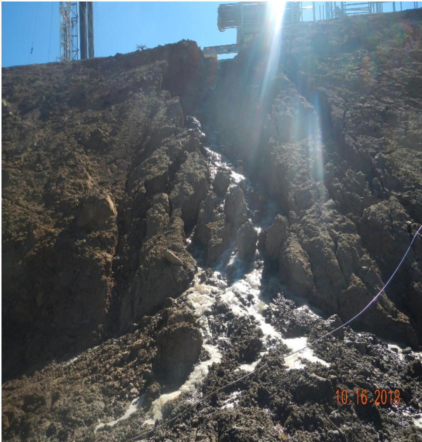
Photo#2: View from base of slope of failed BMP area 10/16/18.
