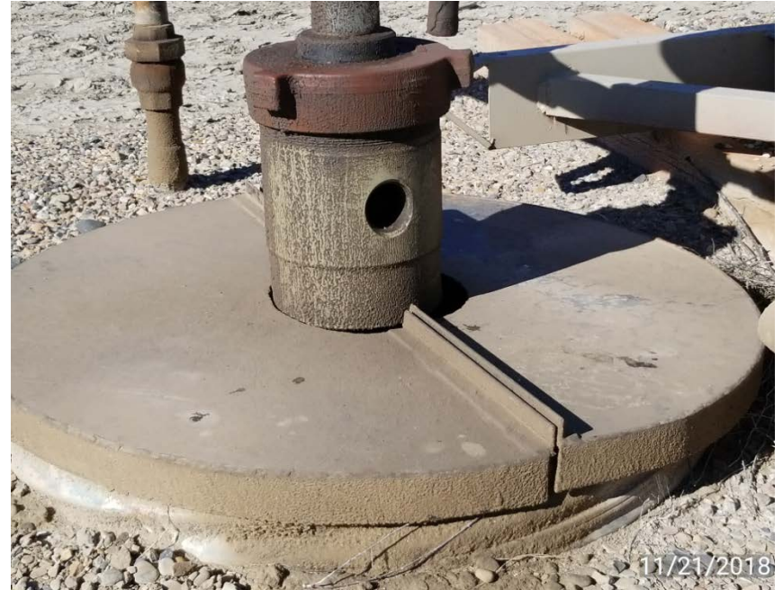
Photo 2. Well head with casing open to atmosphere.
