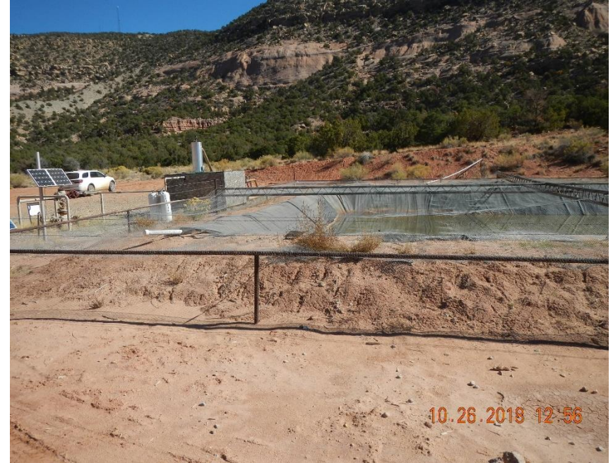
Pit Facility ID #112976 with leak detection system visible.
