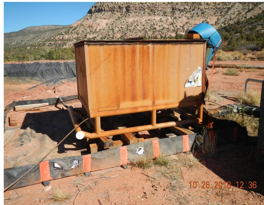
Produced water AST in secondary containment. Two approximately 900 gallon tanks are in use until repairs to pit are complete.
