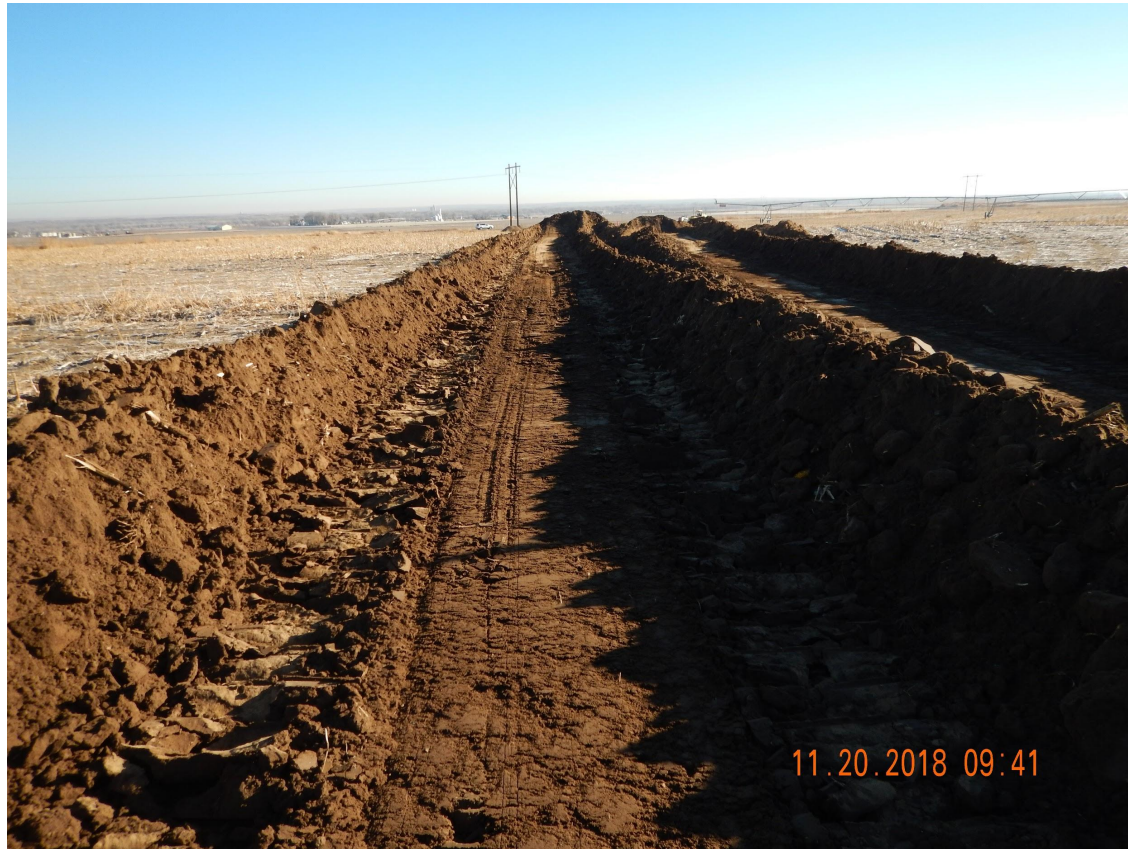
Photo 3. Photo taken from the initial topsoil salvage area, facing East. COGCC Staff is observing that all topsoil is being salvaged. Operator stated that topsoil would be salvaged from the entire disturbance area to a depth of 12”.
