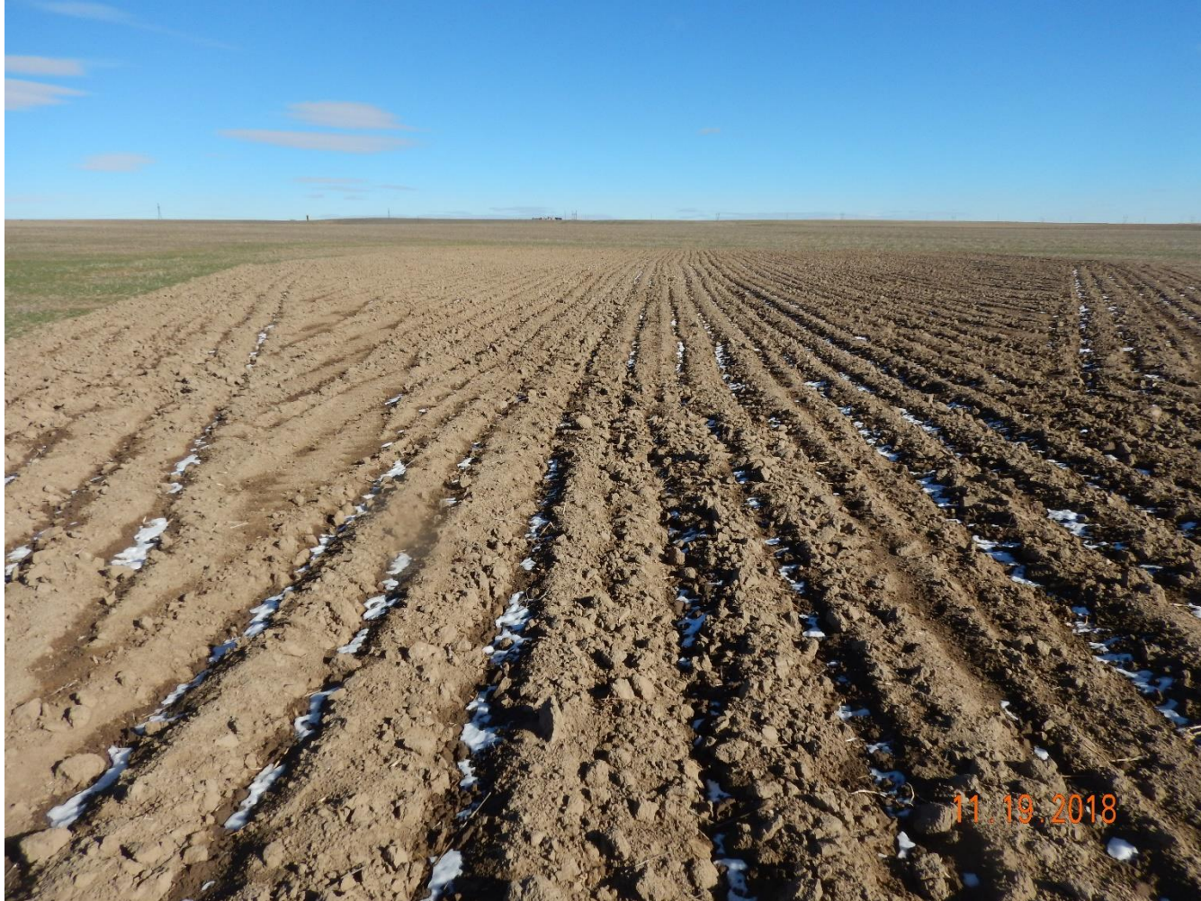
Photo 5: Photo taken from the location, facing east. Photo shows overview of the location. Photo shows reclamation does not appear to have been conducted in accordance with 1000 series reclamation requirements; 1004.a requires compaction alleviation to be conducted by cross-ripping to a depth of 18 inches. Location has not been cross ripped. Compaction concerns remain evident.
