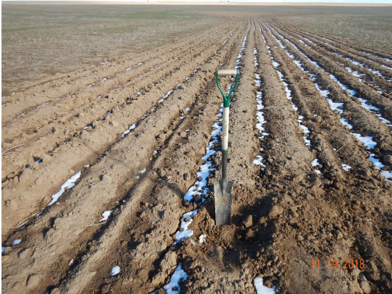
Photo 2: Photo taken from the access road, facing east. Photo shows inspector tested the location for compaction. Photo shows inspector found compaction zones a few inches sub-surface within areas of the road that were not cross-ripped.
