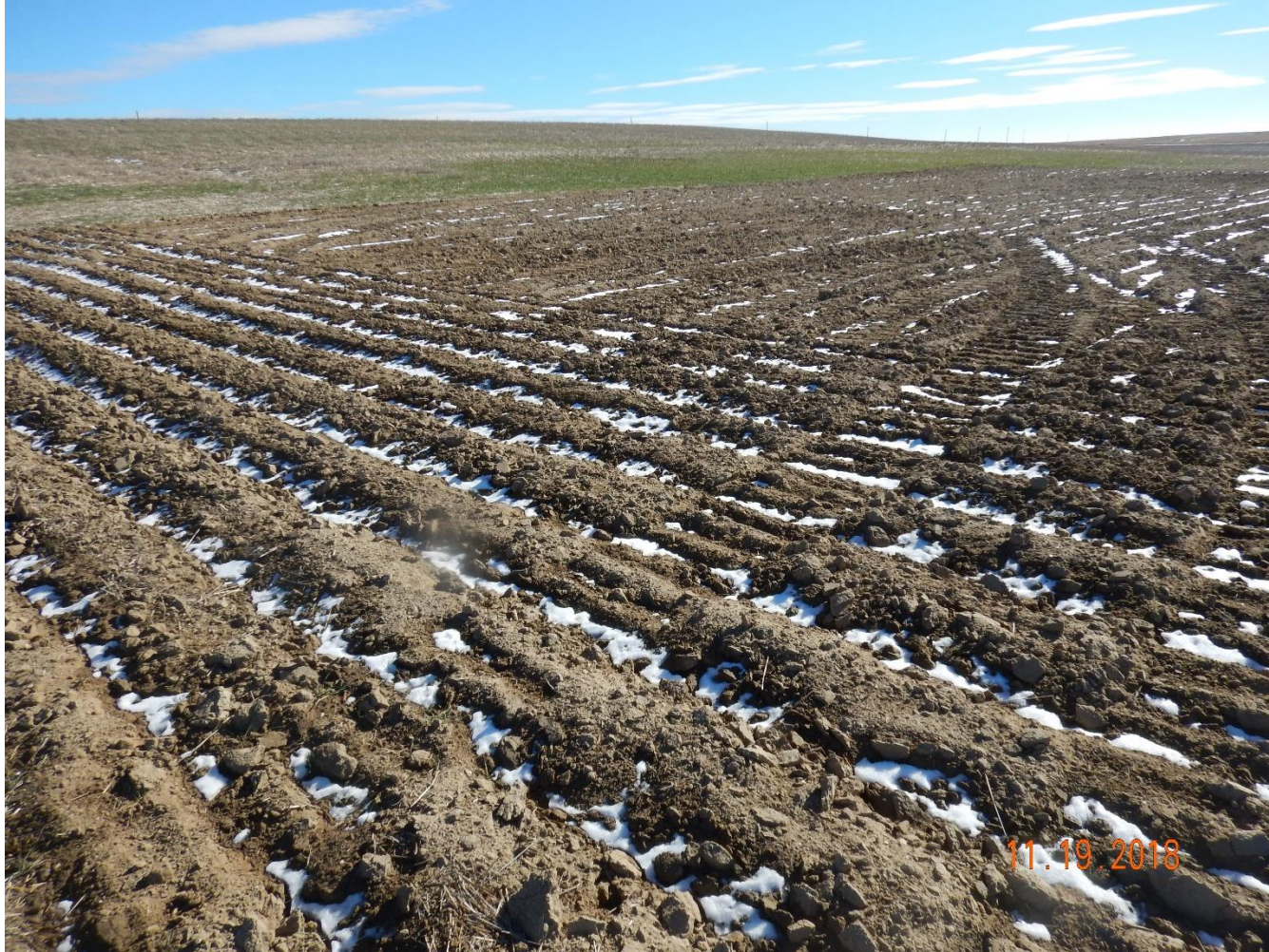
Photo 1: Photo taken from the north end of the location. Photos 1-3 provide an overview of the location from east, to south, to west. Photos also show that additional reclamation appears to have been conducted, however reclamation does not appear to have been conducted in accordance with 1000 reclamation requirements; 1004.a requires compaction alleviation to be conducted by cross-ripping to a depth of 18 inches. Location has not been cross-ripped. Compaction concerns remain evident.
