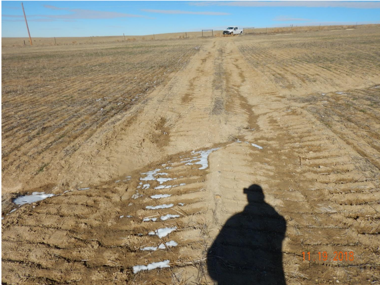
Photo 7: Photo taken from the access road, facing north. Photo shows access road. Unable to find evidence that compaction alleviation has been conducted in accordance with 1004.a. Access road also does not appear to have been re-contoured or re-graded. Photo also shows erosion degradation on road.
