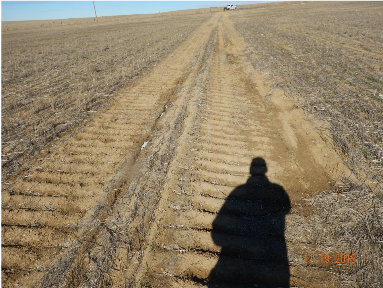
Photo 6: Photo taken from the access road, facing north. Photo shows access road. Unable to find evidence that compaction alleviation has been conducted in accordance with 1004.a. Access road also does not appear to have been re-contoured or re-graded.
