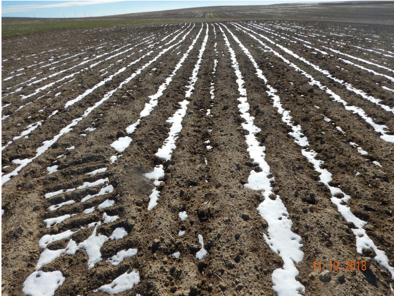
Photo 4: Photo taken from the location, facing south. Photo shows location appears to have been ripped in one direction. 1004.a requires compaction alleviation to be conducted by cross-ripping to a depth of 18 inches. Location has not been cross-ripped. Compaction concerns remain evident.
