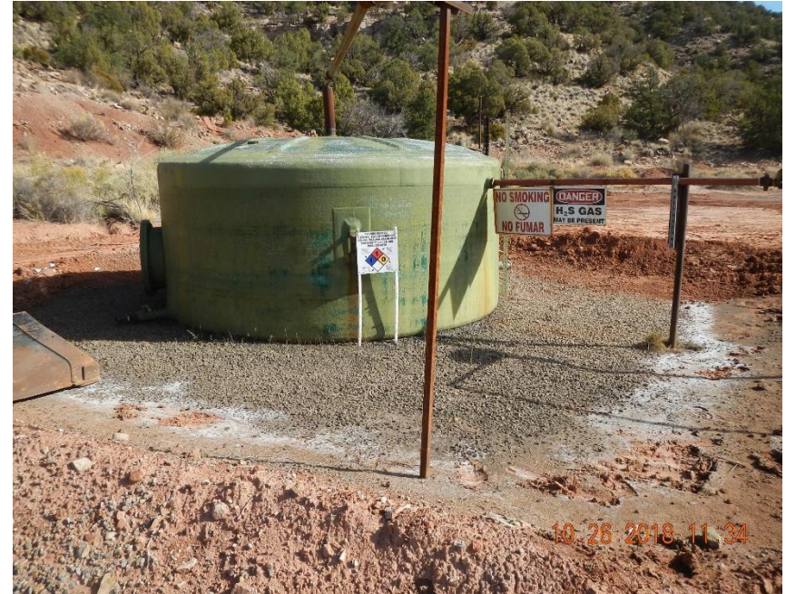
White residue present within secondary containment berm.
