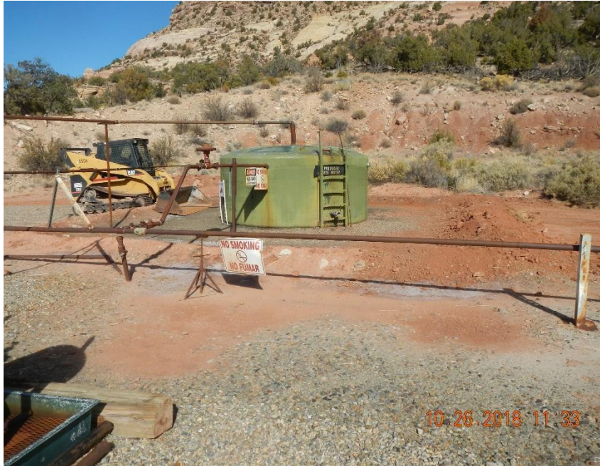
2,500 gallon fiberglass produced water AST where release occurred.
