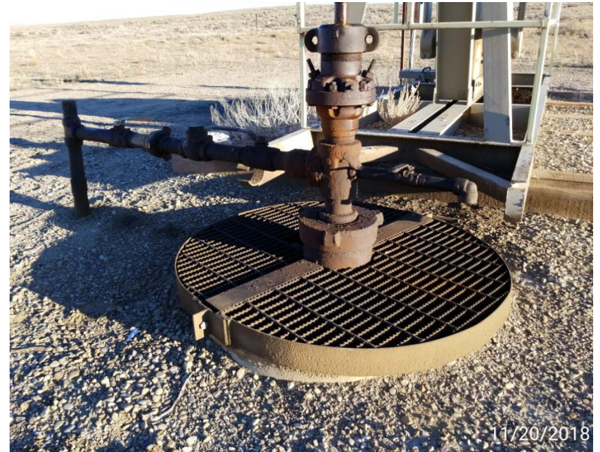
Photo 2. Wellhead. Not venting. No valve below cellar. Valve above cellar closed.
