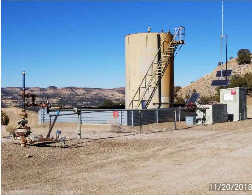
Photo 1. Location looking west.
