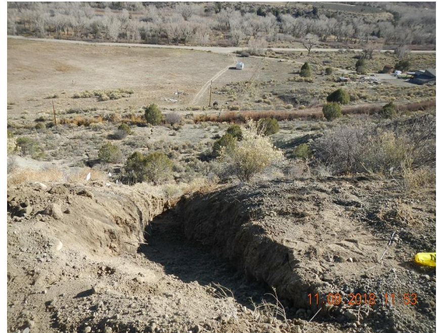
Initial excavation of flow path.
