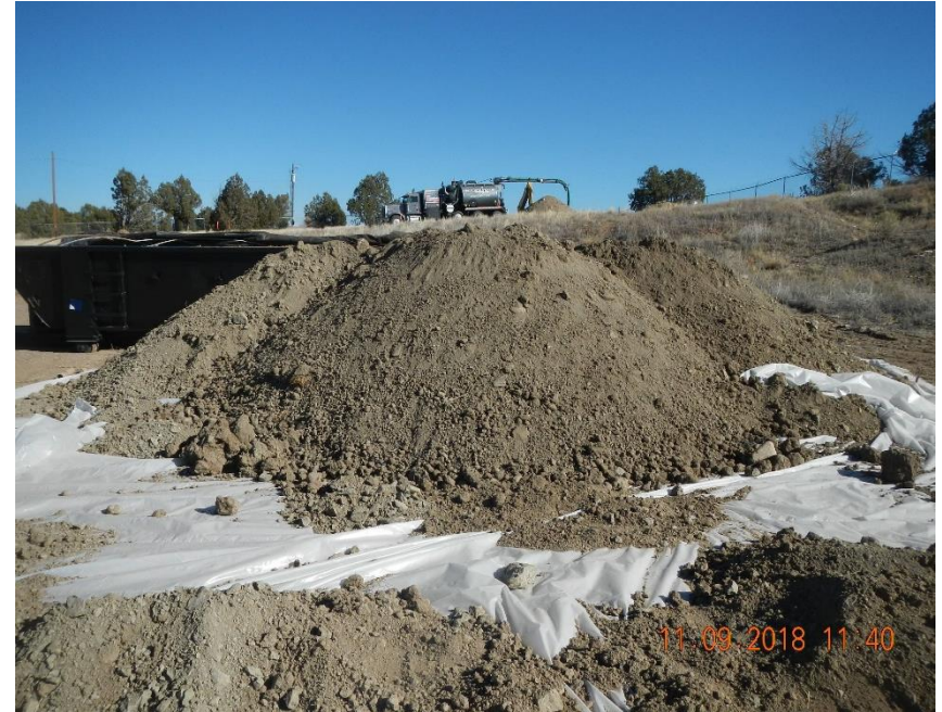
Soil excavated from pipeline ROW.
