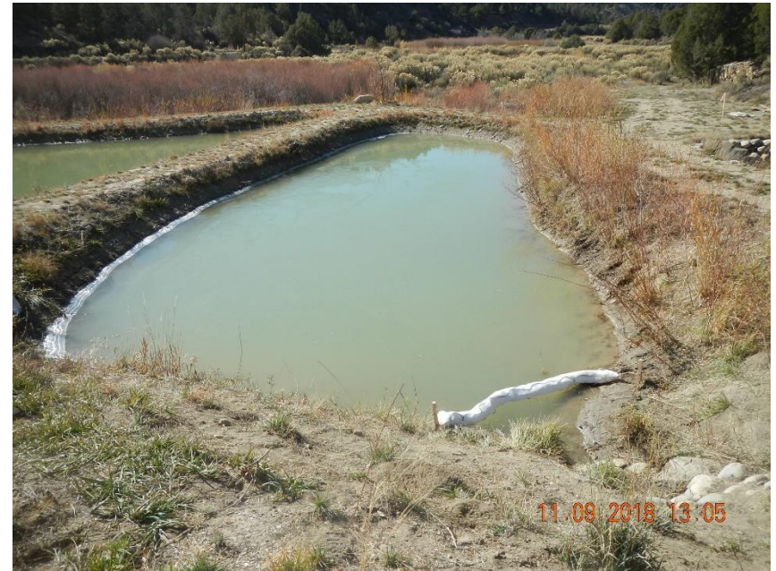
Boom in Pond #4 near inlet.
