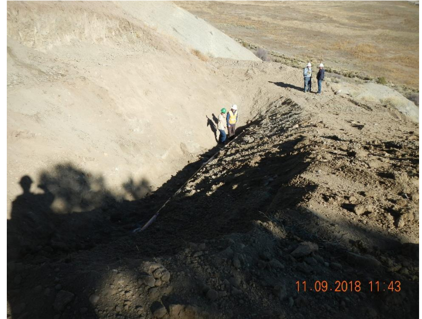
Excavated 6" fiberglass produced water pipeline.
