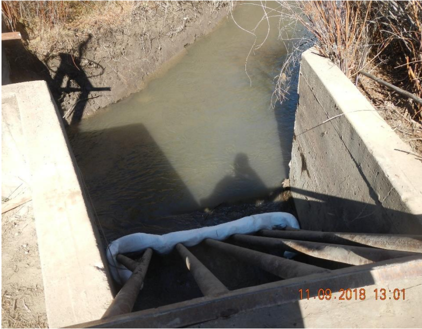
Boom across High Flume Canyon siphon inlet.
