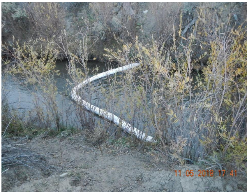
Absorbent boom below Point of Contact with irrigation ditch.
