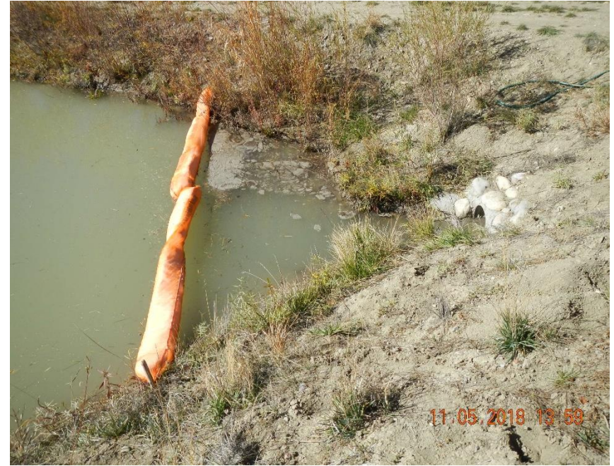
Inlet to Christine's Pond with absorbent booms in place.
