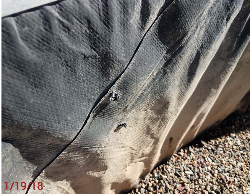
Location Photo #5, Holes in battery liner
