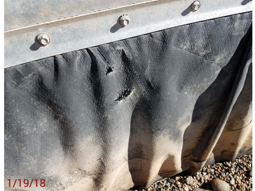
Location Photo #4, Holes in battery liner.
