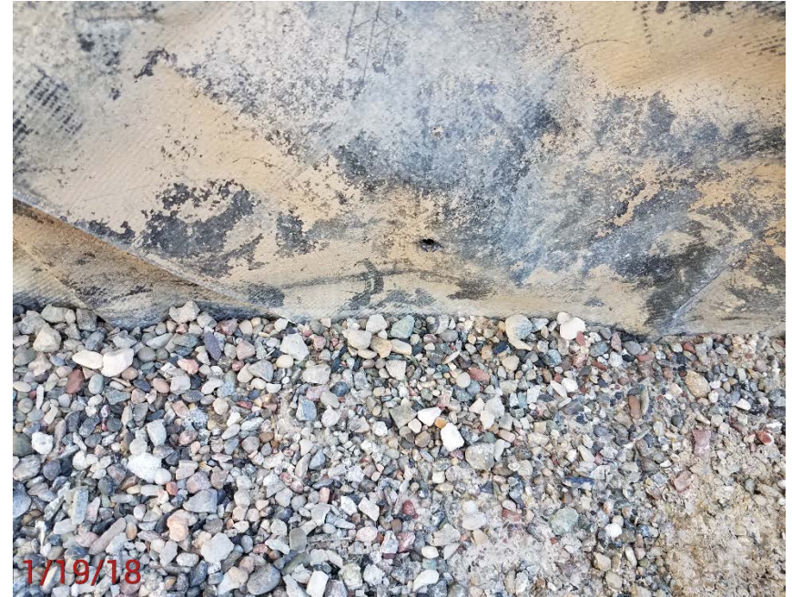
Location Photo #6, Holes in battery liner.
