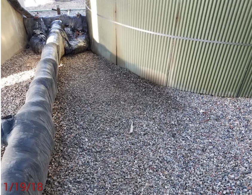
Location Photo #3, Oily stained rock in battery containment.
