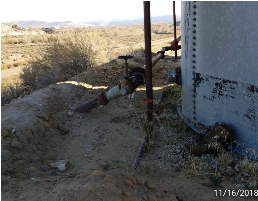
Photo 3. Insufficient berm capacity due to short berm on north side.
