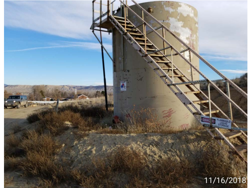
Photo 6. Berm capacity insufficient.
