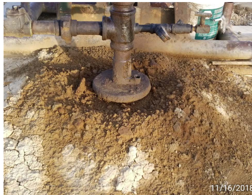
Photo 2. Oily waste around wellhead.
