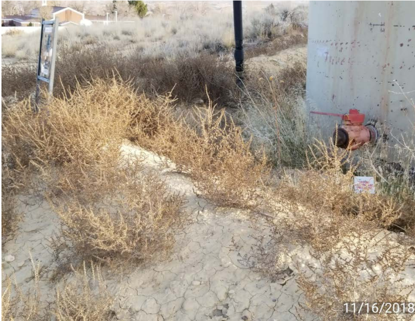
Photo 3. Weeds on and inside berm.
