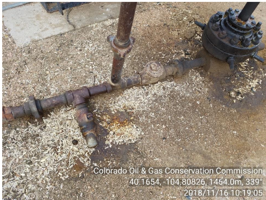
PHOTO 3: STAINED SOIL UNDER VALVE & AROUND WH
