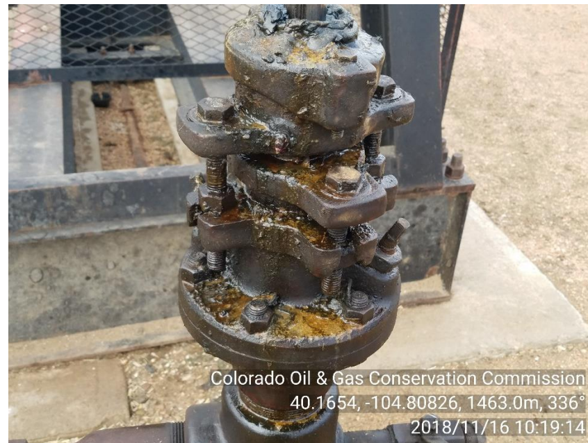
PHOTO 4: PLUNGER ROD PACKING LEAKING
