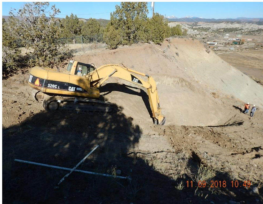
Initial excavation work on the pipeline ROW at the release point. Work is being done to expose and inspect the failed 6" fiberglass PW transfer line. View looking North.
