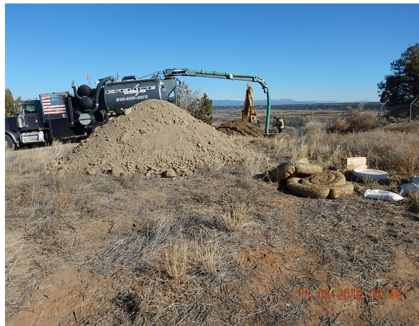
Hydro-excavation in progress at the valve can located approximately 115' SW of the water transfer line failure. Excavation in progress on the ROW downslope from the valve can.
