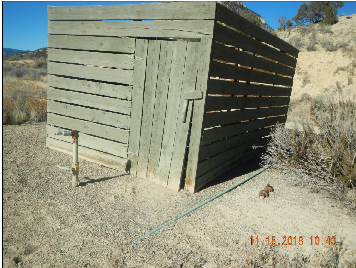
Unused equipment at well.
