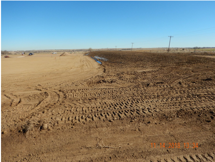
Photo 9. Photo taken from the southwestern perimeter of the location, facing East. Photo illustrates the southern topsoil stockpile that has been temporarily stabilized with equipment tracking.
