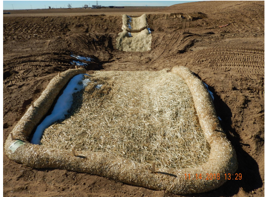
Photo 2. Photo taken from the northeastern perimeter of the location, facing West. Photo illustrates a sediment trap with a temporarily stabilized outlet.
