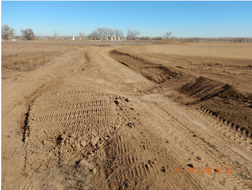
Photo 7. Photo taken from the northwestern perimeter of the location, facing North. Photo illustrates a retention area installed in conjunction with the ditch and berm BMP.
