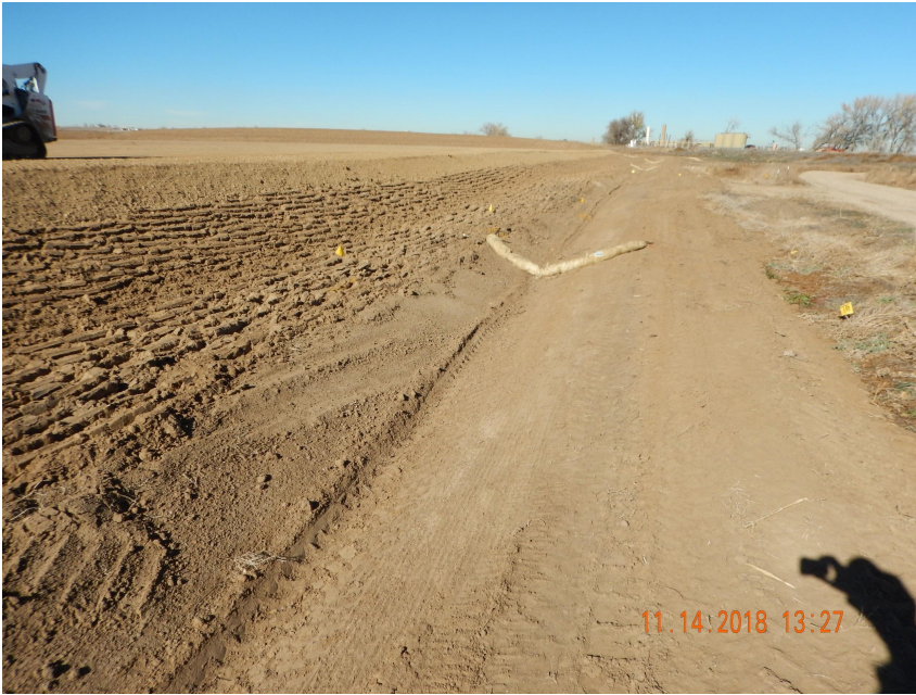
Photo 1. Photo taken from the southeastern perimeter of the location, facing North. Photo illustrates a ditch and berm BMP that has been installed around the entire perimeter of the location in conjunction with other BMPs.
