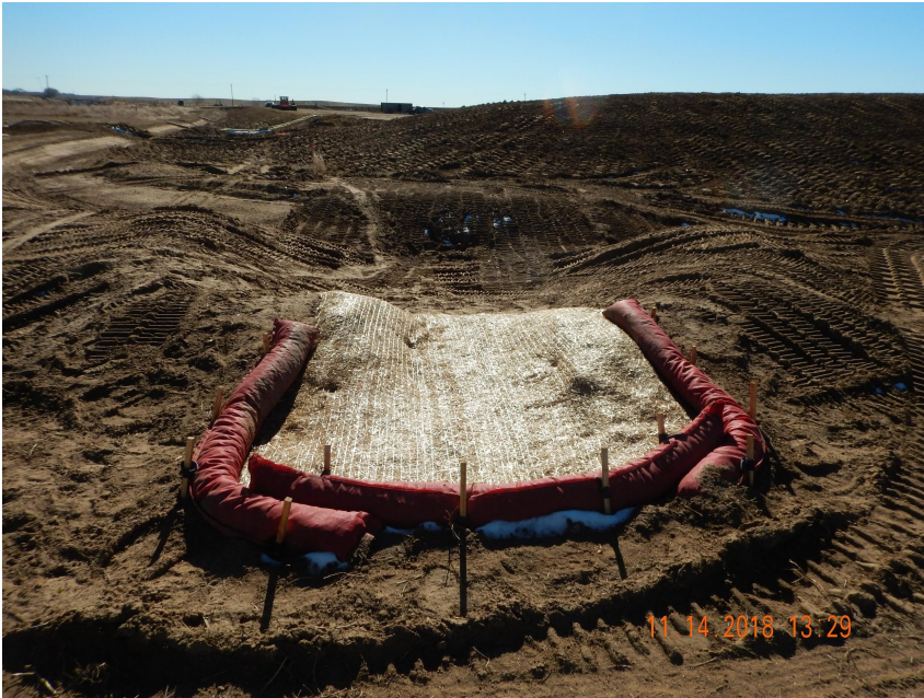
Photo 3. Photo taken from the northeast perimeter of the location, facing South. See comments under Photo 2.
