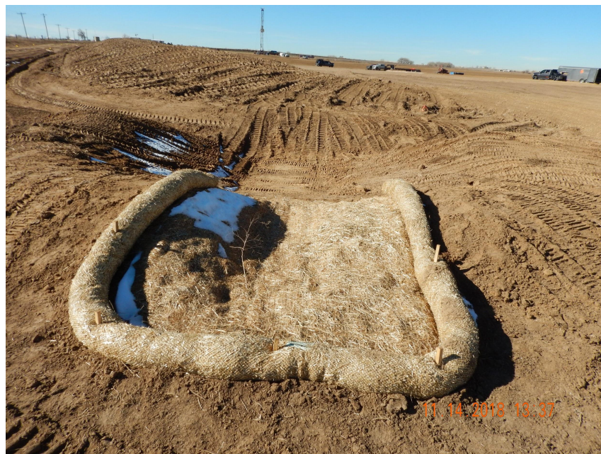
Photo 14. Photo taken from the southeast perimeter of the location, facing West. See comments under Photo 2.
