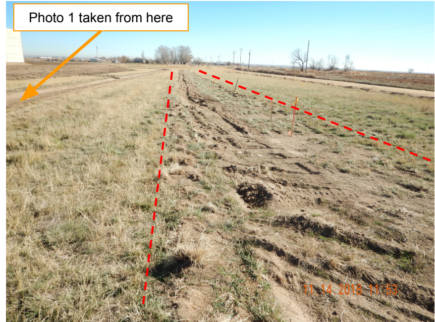
Photo 2. Photo taken from the southern perimeter of the location, facing East. Photo illustrates the start of a perimeter BMP disturbance. BMP was moved more north. Operator will be responsible for recontouring the said disturbance and comply with other Rule 1004 standards (i.e., vegetation).
