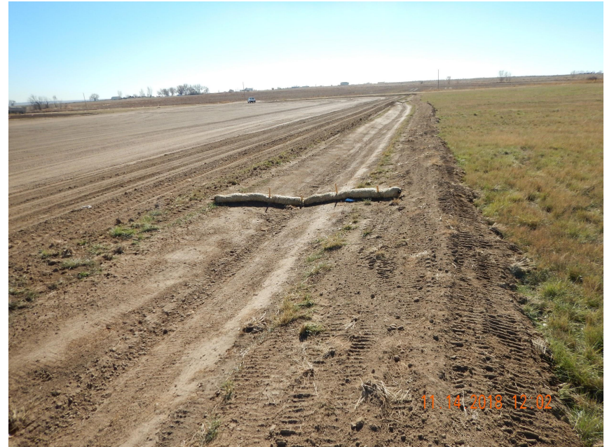
Photo 10. Photo taken from the western perimeter of the location, facing South. See comments under Photo 1. Straw wattles have been installed in conjunction with the western ditch and berm BMP.
