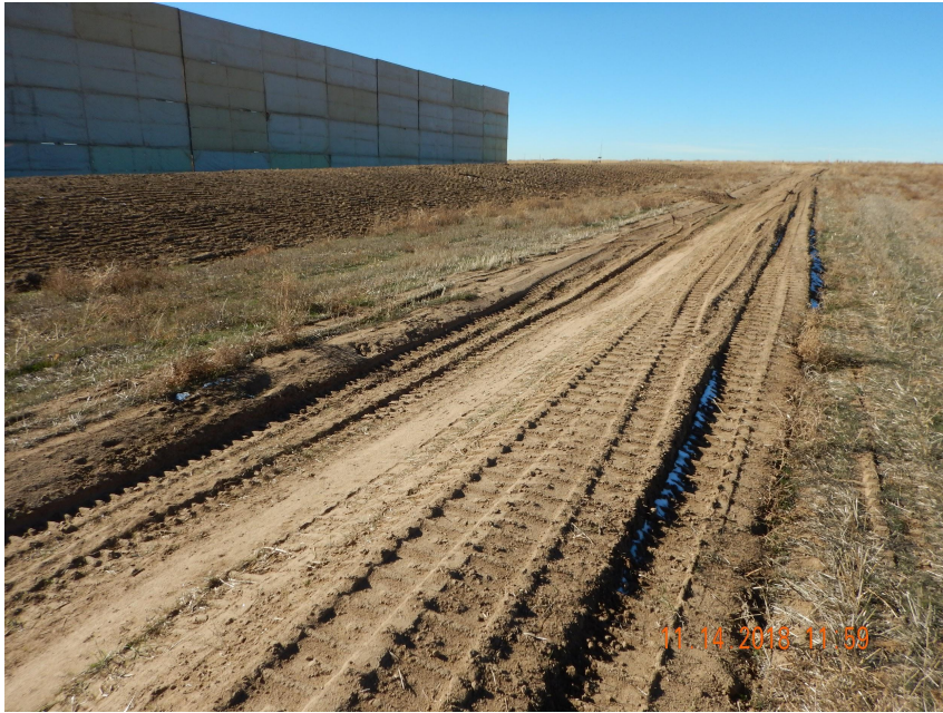
Photo 7. Photo taken from the northeastern perimeter of the location, facing West. Photo illustrates the ditch and berm BMP, and the temporarily stabilized topsoil stockpile.
