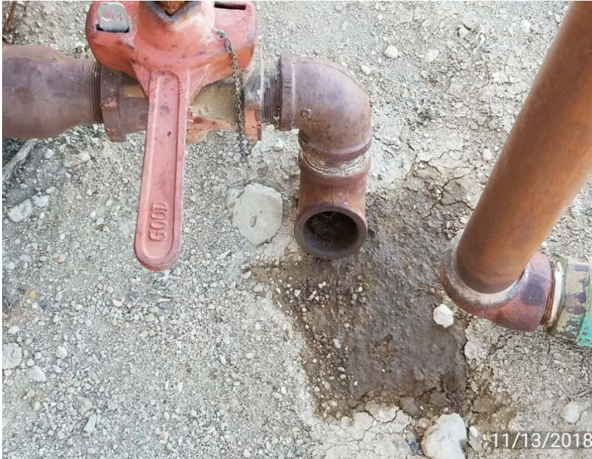
Photo 5. Oily waste from tank valve.
