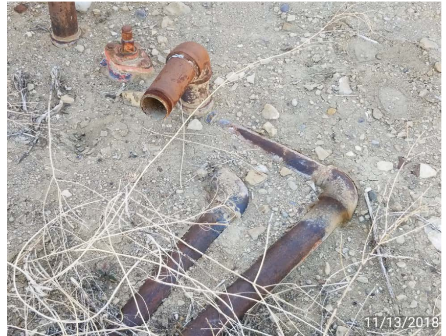
Photo 8. Riser not capped or locked out tagged out
