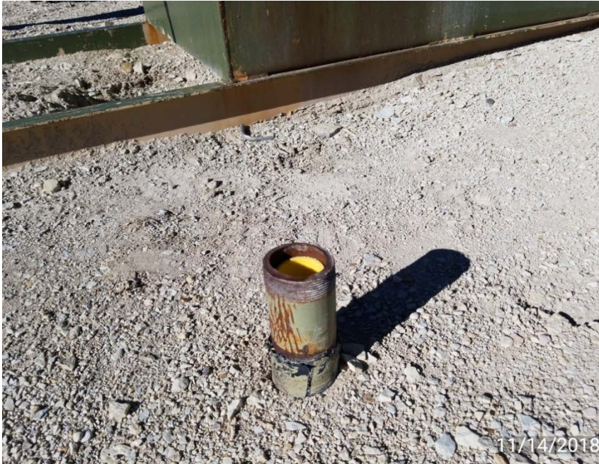
Photo 3. Riser not capped or lock out tagged out.
