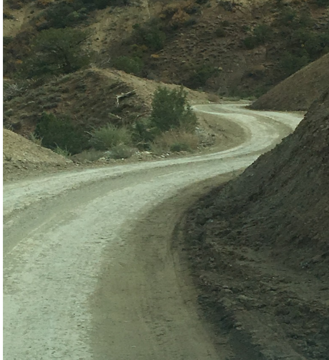
Photo 1. Access road leading to the MV 60-8D well pad. Surveyed 17% grade.
