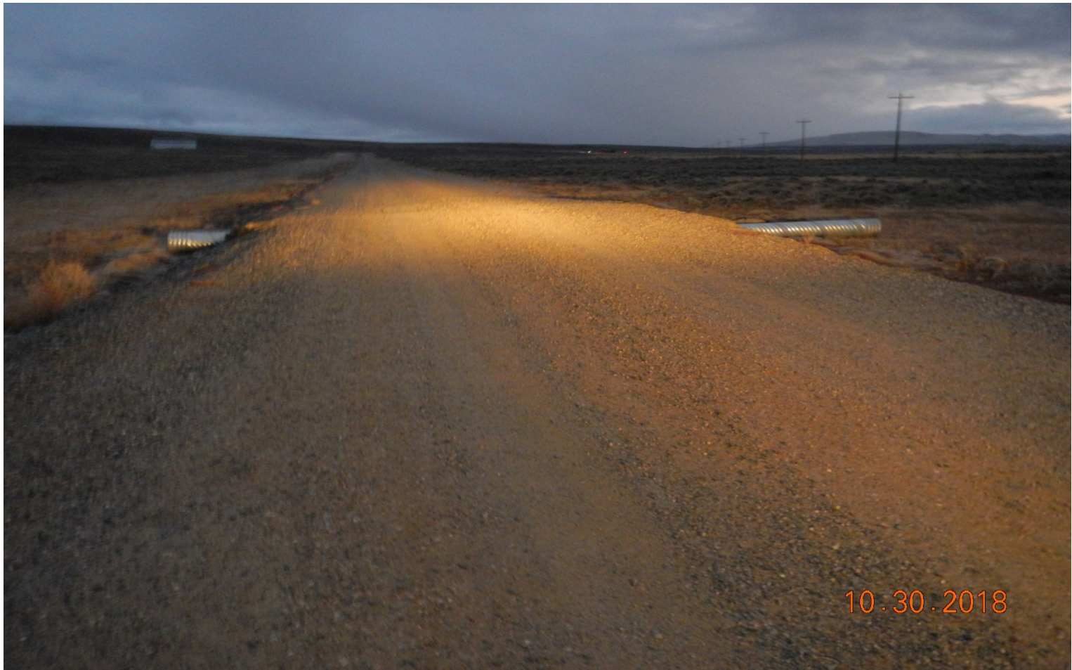
Photo#3: Culverts have been installed along access road..
