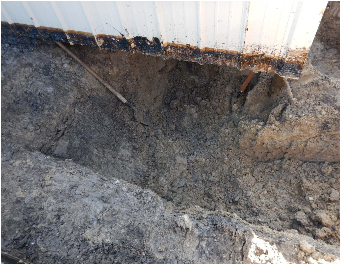
Flowline excavation inside containment below treater house at tank battery.
