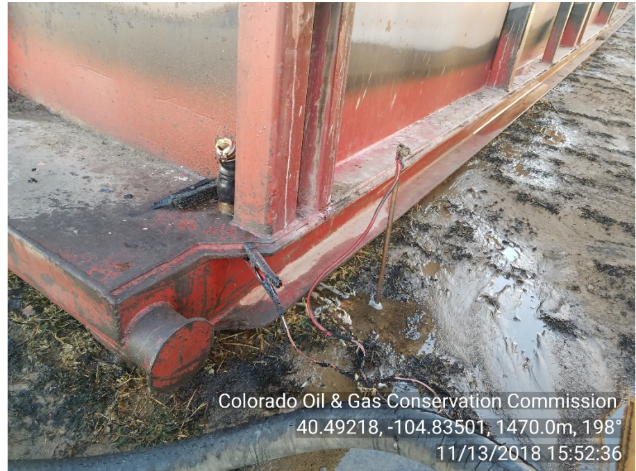
Grounding rod on north tank
