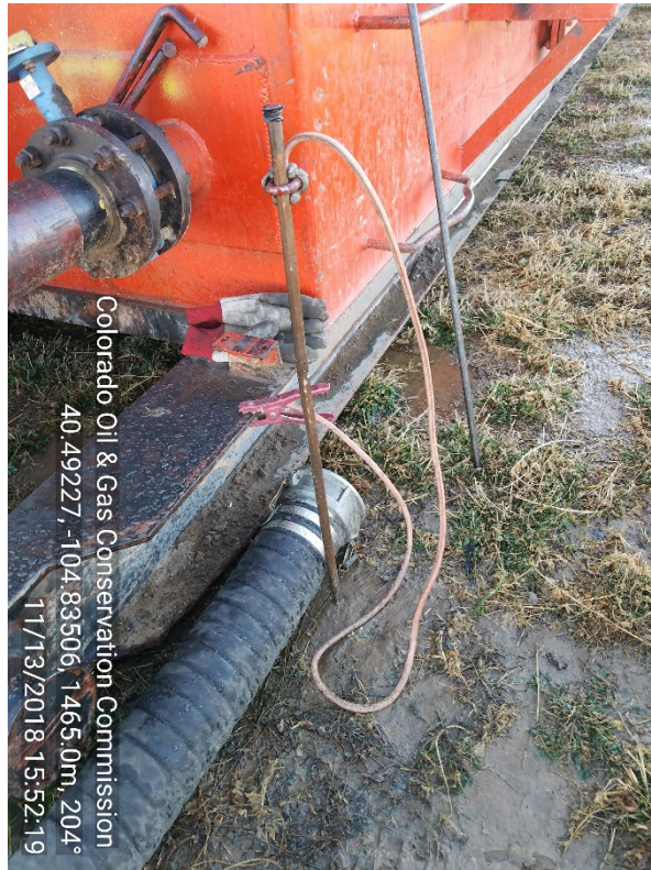
Grounding rod on south tank
